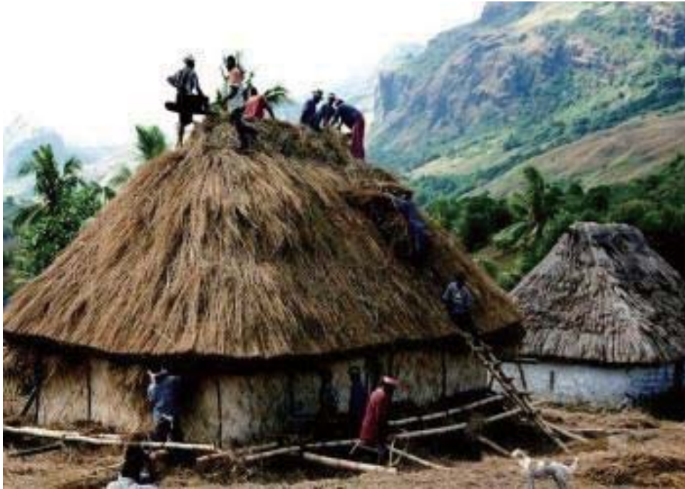
Revitalization of traditional bure building
